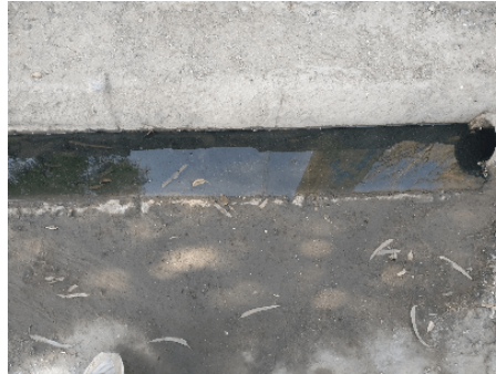
Figure 3 A pipe connects household sewage to a street. Source: Photography by the author.
