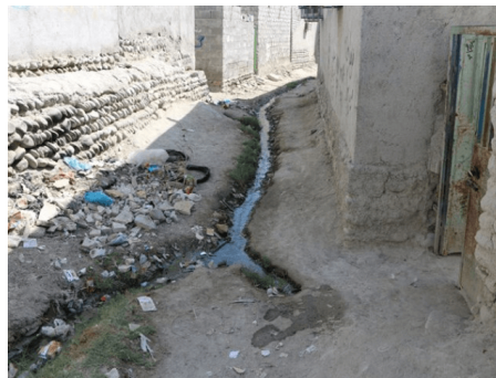
Figure 4 Sewage enters from homes into the creek in the middle of the alley and streets. Source: Photography by the author.
